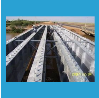
Plate Girders Fabrication
