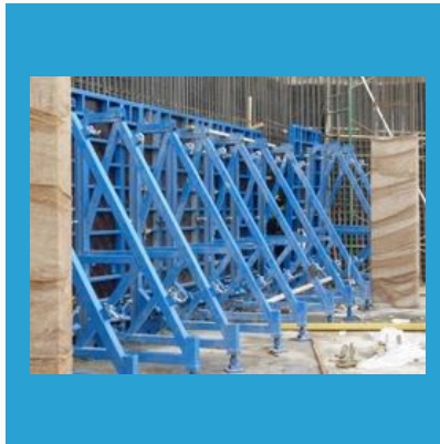
Single Sided Formwork System
