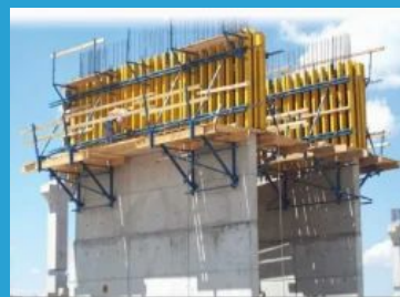
Climbing Formwork & Jump Form
