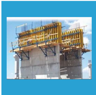
Climbing Formwork & Jump Form
