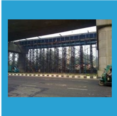
Pier and Deck Slab Shuttering
